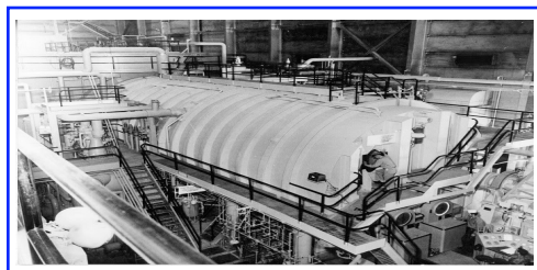
The interior of the Submarine 1st Generation Westinghouse facility located at the Naval Reactors Facility at the U.S. Department of Energy Idaho National Laboratory Site, circa mid-1950s.
