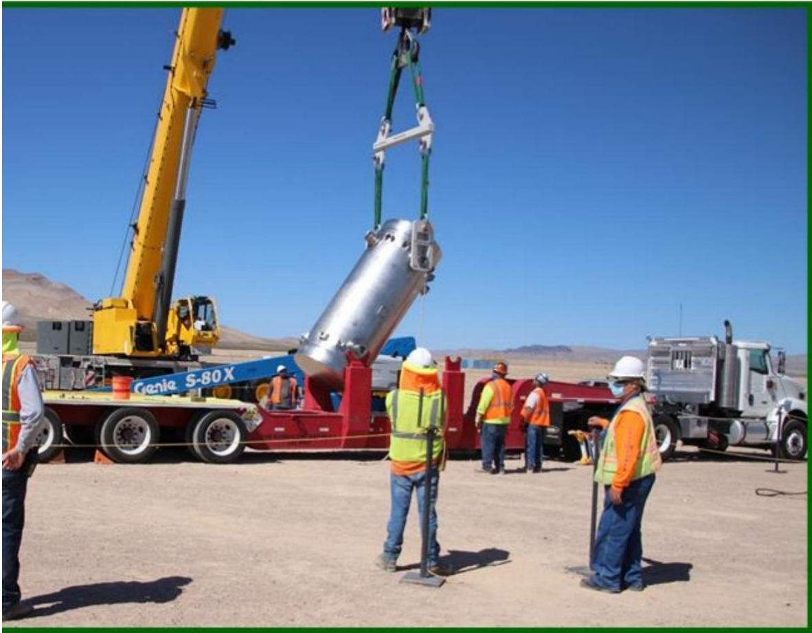
loading TN RAM transportation cask containing Oak Ridge National Laboratory LLW at Nevada National Security Site Area 5
