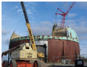
Decontamination and Decommissioning
