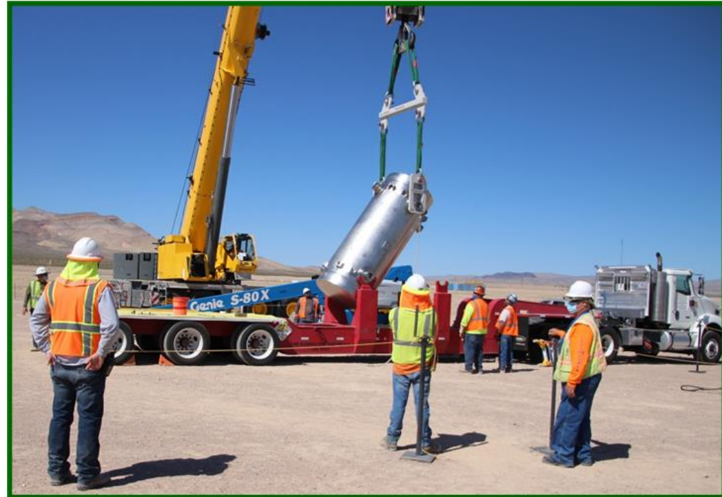
Offloading TN RAM transportation cask containing Oak Ridge National Laboratory LLW at Nevada National Security Site Area 5
