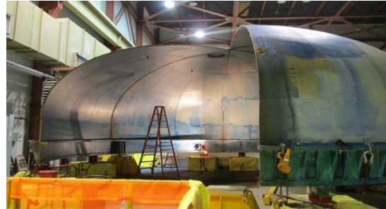
Oyster Creek Drywell Head Segmentation
