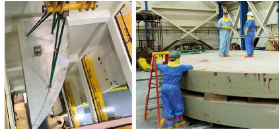
Oyster Creek Reactor Containment Shield Piece Cutting / Removal
