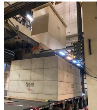
Storage in Concrete Box until ready for Offsite Transport
