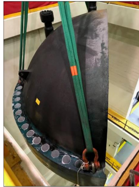
Oyster Creek Reactor Head Segmented
