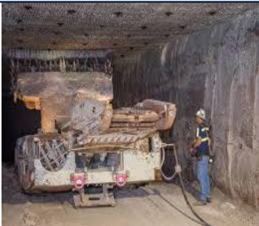
Mining in WIPP underground provides needed capacity to support DOE missions.
