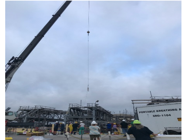
Photo 1: DWPF recycle wastewater retrieval from Tank 22 using sampling vessel and a large crane.
